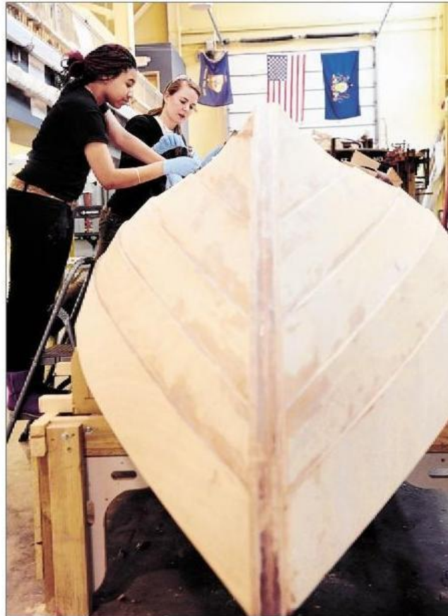
Dazhane Roberts, 17, left, of Erie, and Jodi Carpenter, maritime educator with the Bayfront Maritime Center, apply a sealant to the panels of a 22-foot skiff.
